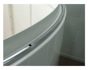
turn, working around the dome from the starting point. If necessary, the last length of track may need to be trimmed with a hacksaw to fit.
