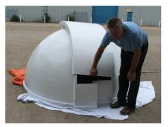
Overlap the dome quadrants at the front (see picture below) and position the lid on to the dome top and carefully locate the guides into the recessed track. When all 4 guides are in place on the track, carefully slide the lid to the back of the dome and silicone and bolt together the front section of the dome quadrants. Care must be taken with the sliding or opening the aperture lid, as it can damage the rear of the observatory dome if allowed to slide back unaided!
